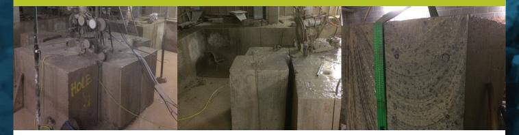
Diaquip needed to provide a fast, long-lasting and cost effective Diamond Wire due to the reinforced concrete blocks needed to be cut as part of this project. It was essential that the wire performed well on reinforced concrete (including steel rebar).
