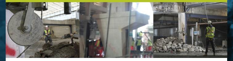
Diaquip needed to provide a fast, long-lasting and cost effective Diamond Wire due to the large quantities used on the project. It was essential that the wire performed well on reinforced concrete (including steel rebar).
