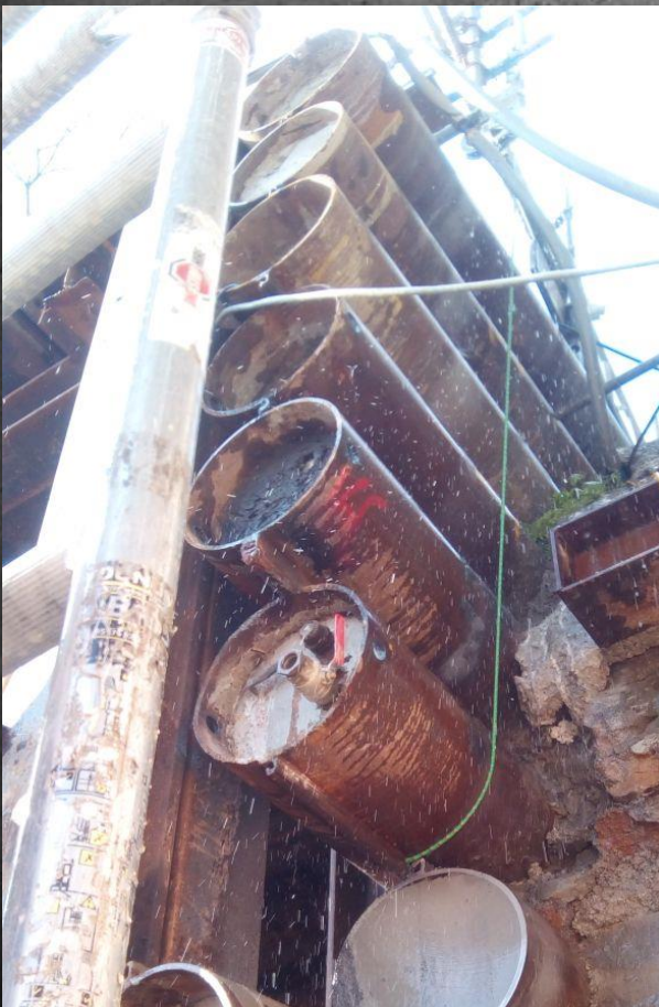
DQ5 wire slicing through Steel Grout Filled Piles!
